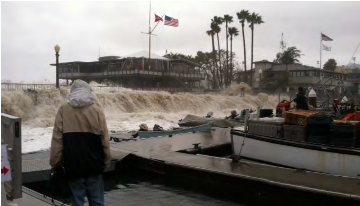
Figure 3 Overtopping at the Southwest Corner of the Harbor Breakwater in March 2014
