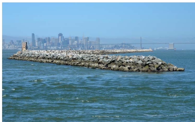
Figure 14: Fully armored breakwaters, such as this one in Alameda, can help reduce flooding from coastal storms but may make conditions worse elsewhere Source: Alameda Point Environmental Report
