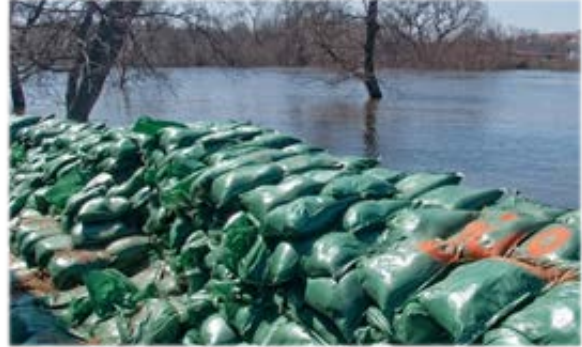
Figure 17: A ready supply of sandbags helps make it easier for City staff to construct flood barriers before a storm occurs
