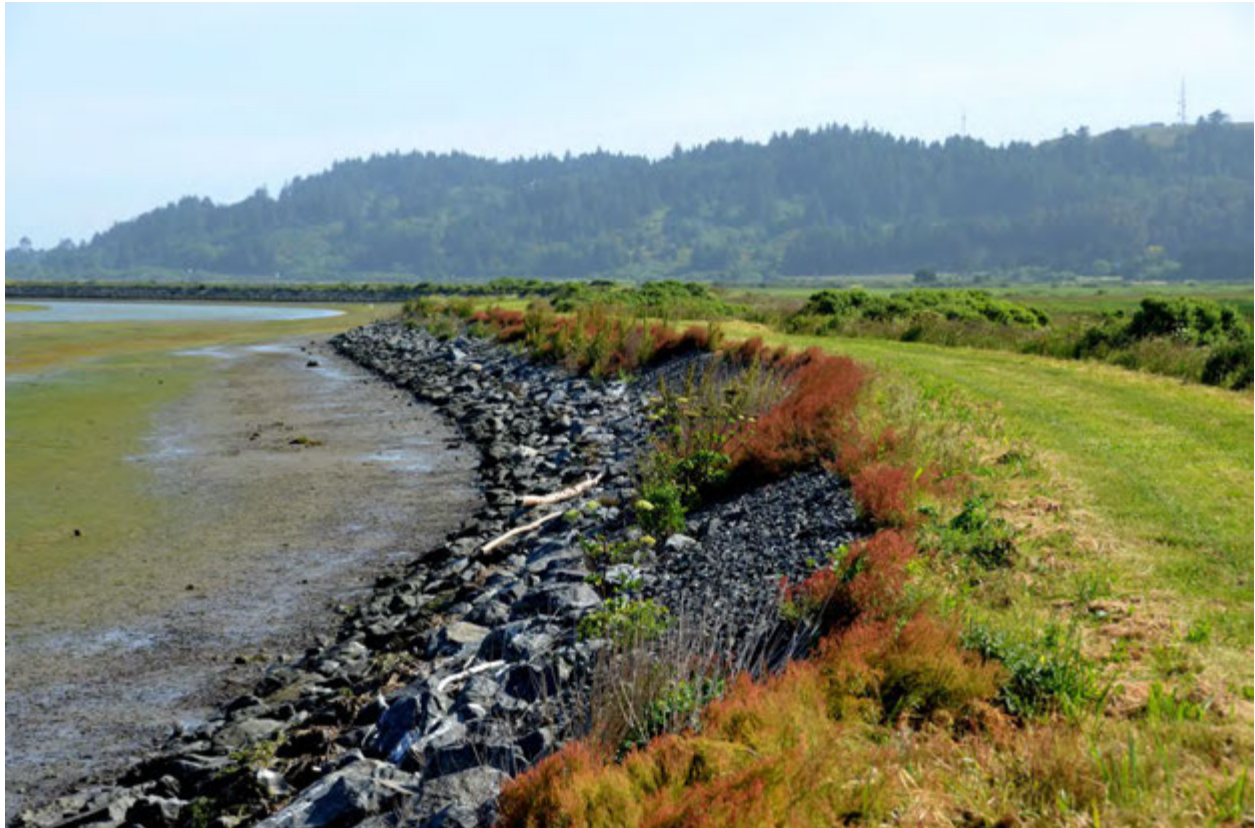
Figure 11. Hookton Slough on South Bay is an example of an earthen dike with rock revetment and roadway that is being maintained.
