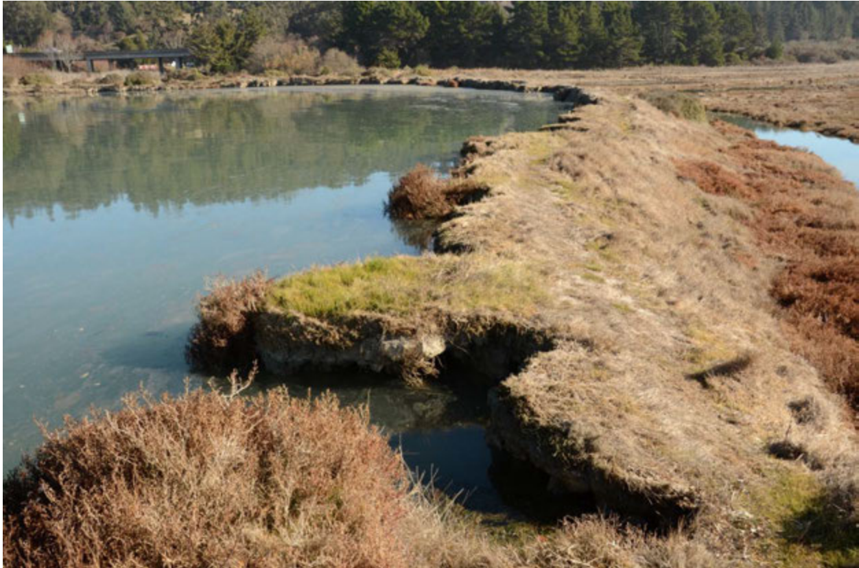
Figure 3. An example of a diked shoreline segment rated highly vulnerable and at risk of breaching that could tidally inundate former tidelands.
