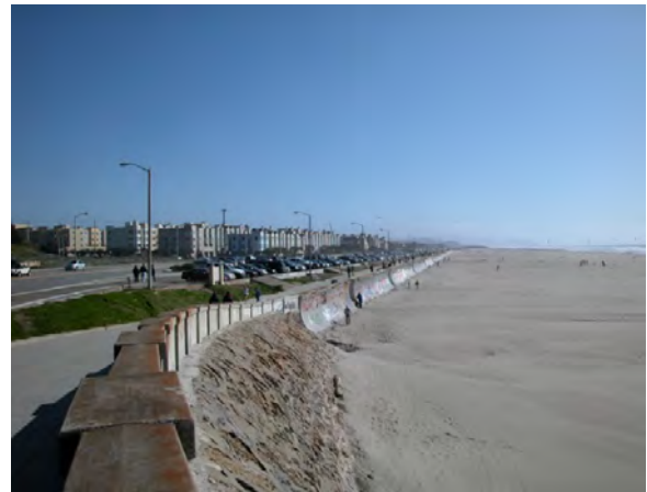
Example of hard shoreline protection. Portions of San Francisco’s Ocean Beach is partially armored by a concrete seawall and supplemented with regular beach nourishment.
