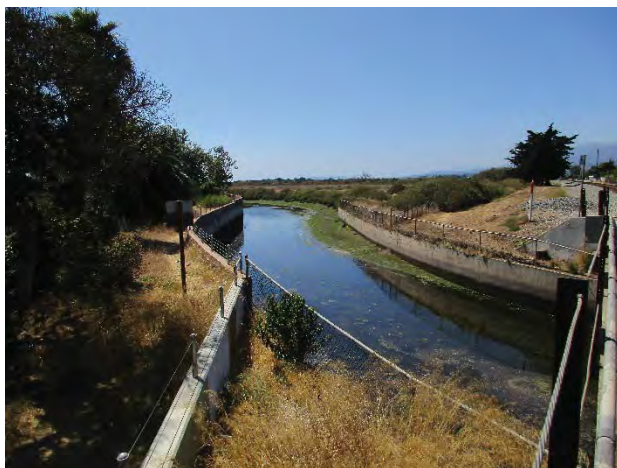
Formerly natural bottom Franklin Creek has been channelized within a concrete box channel to convey stormwater runoff to Carpinteria Salt Marsh. When combined with storm surges, Franklin Creek can contribute to localized flooding.
