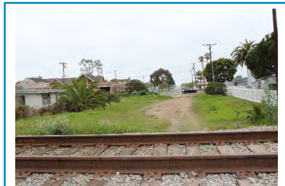
The UPRR tracks near Ash Avenue are raised about four feet above the roadway and could protect landward infrastructure from flooding with up to approximately 2 feet of sea level rise.
