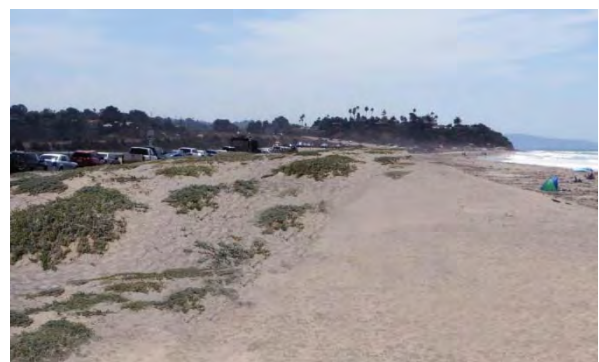
Dune concept for the Cardiff State Beach living shoreline project, which would utilize dunes instead of rock revetments to ensure protection for the adjacent roadways. Photo Source: California Coastal Conservancy.
