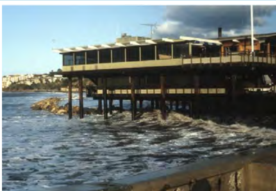
Example of accommodation approach. The Santa Barbara Yacht Club is elevated above the shoreline using caissons, water-tight pier structures. The parking lot and beach flooded during the 1983 El Niño event. Photo credit: Gary Griggs
