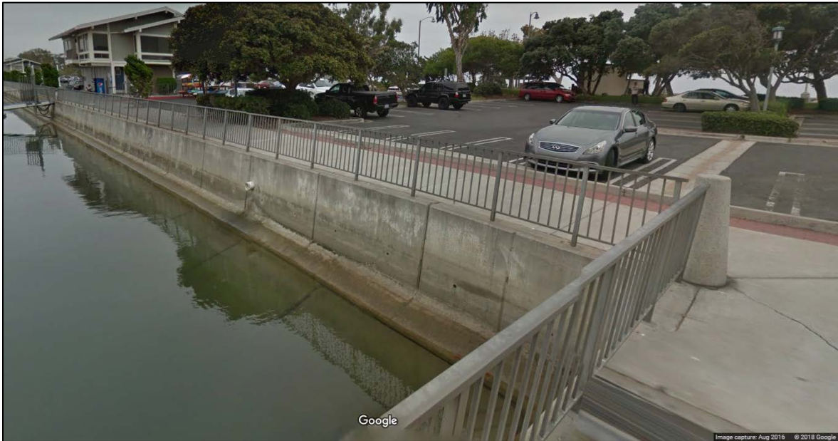
Figure 2-3: Typical Edge Condition for Dana Point Harbor Comprising a Concrete Bulkhead with Rail Fencing (Google Streetview, 2016)
