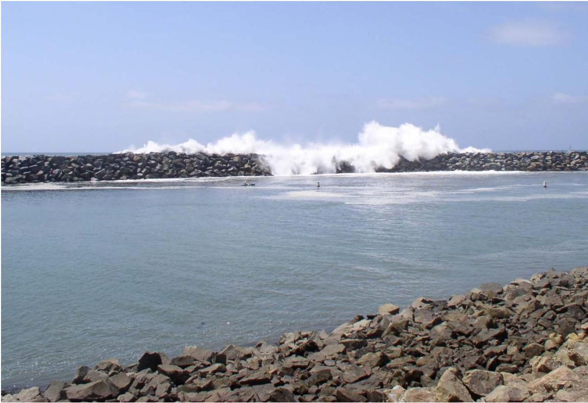
Figure 4-3: Overtopping of West Breakwater in April 2007
