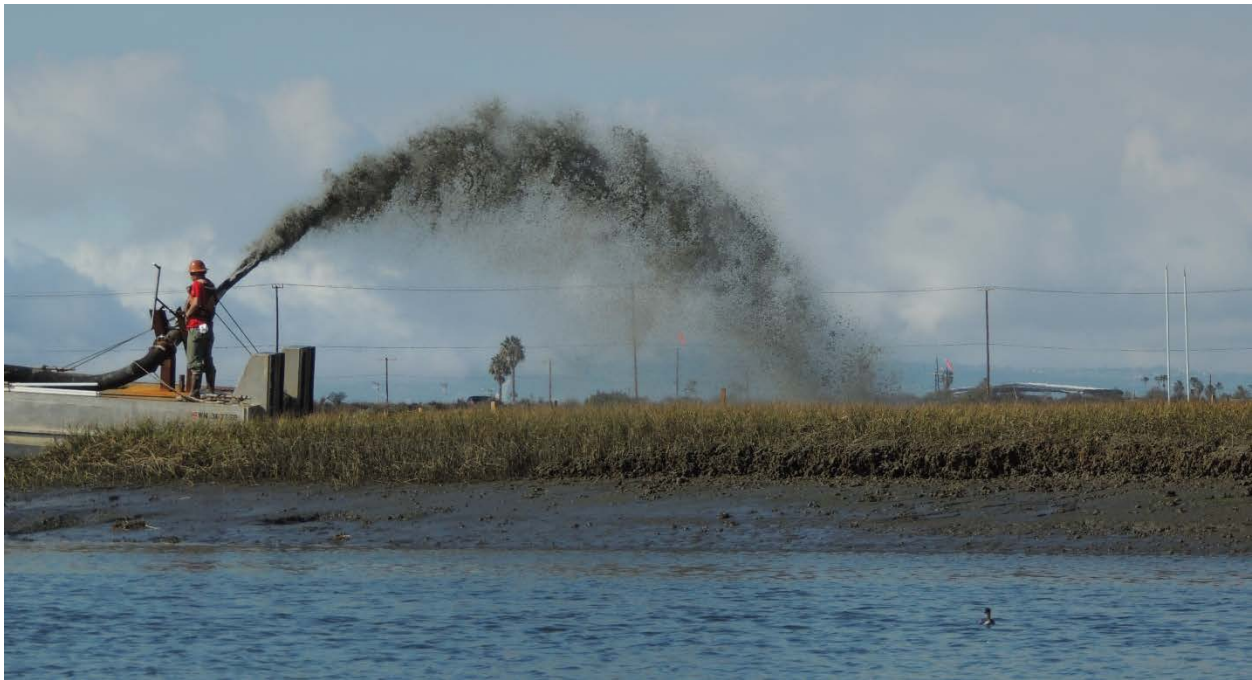
Figure 6-2: Thin-layer sediment placement within the Seal Beach National Wildlife Refuge (M&N, 2016)
